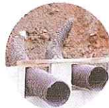
Cool and Warm Air Tubes (Utilizing ground heat from part of the underground area.)
